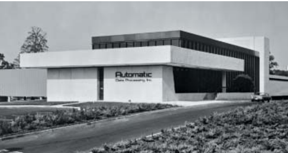
The 405 Route 3 building in Clifton, NJ, was ADP's first, all-new structure. For nearly a decade-and-a-half, it served as ADP's Corporate Headquarters.
